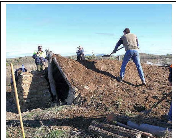
Finished Miner's Dugout
