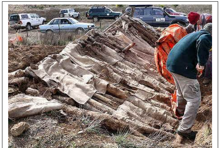
Removing old Miners Dugout Roof
